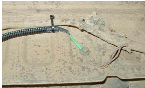
Ground Wire Connected
